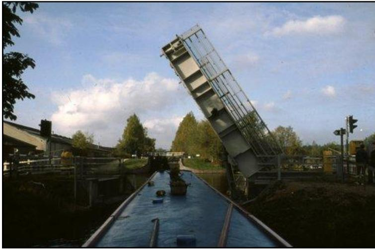
Occasionally you may come across a swing or lift bridge. The photo shows an open lift bridge; swing bridges rotate horizontally on a fulcrum.
