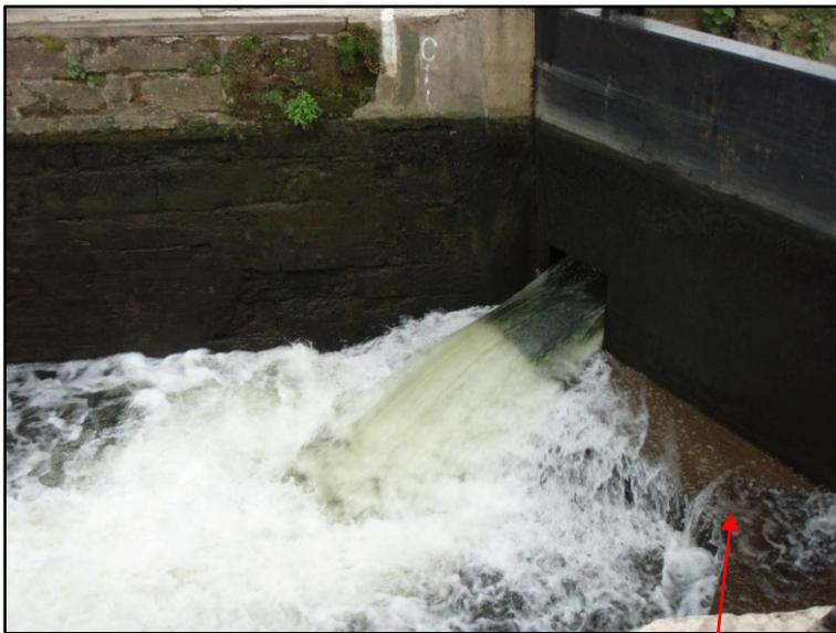
A gate paddle fully open showing the force of water that can enter the lock chamber. The cill can be seen on the right hand side at the base of the gate
