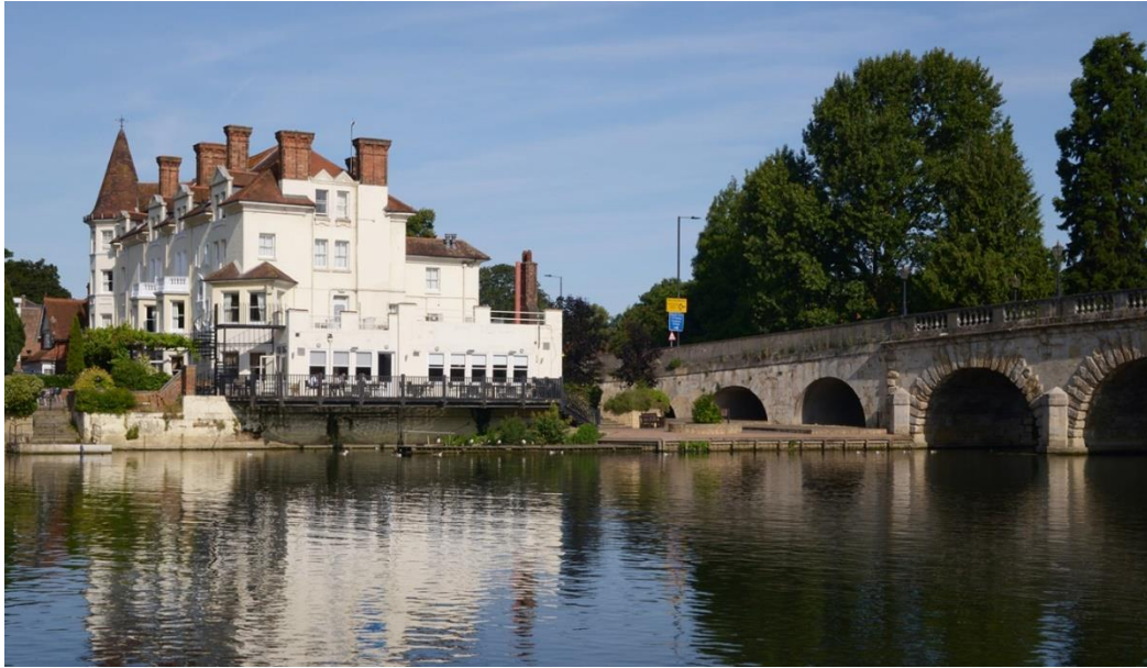
Maidenhead Bridge, designed by Sir Robert Taylor in 1777, and the Thames Riviera Hotel.
