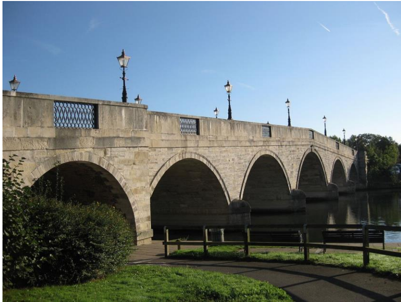
The present Chertsey Bridge, designed by James Paine in the 1780s. The lamps were added in the 1930s
